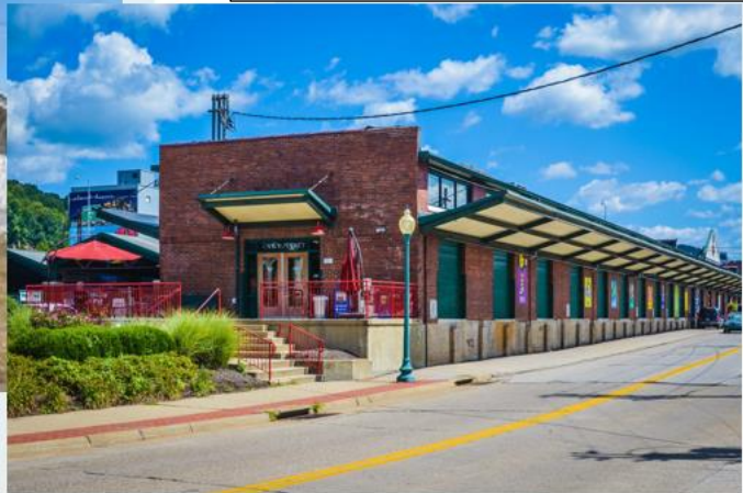
Micro Retailing Opportunities in the Old Depot Building – Public Market, Artisans, Etc.
